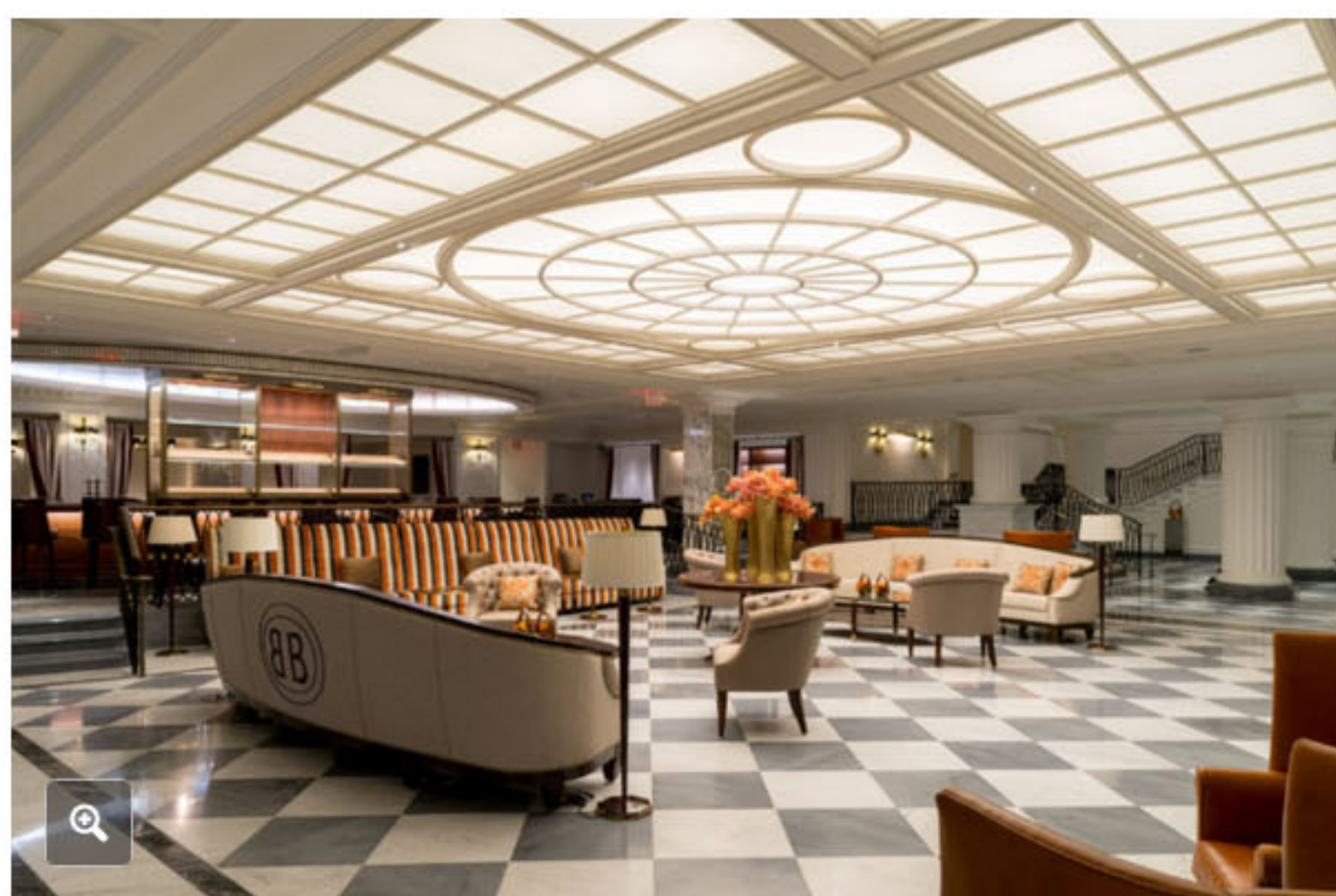
The hotel's renovated lobby. A flat laylight replaced the domed one that had been in the ceiling but no longer fit because of the structural reinforcement needed to support a new ballroom that was installed on the building's second floor. Pablo Enriquez for The New York Times
